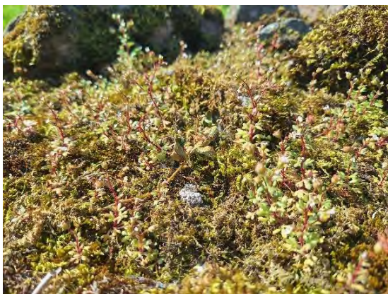
Rue-leaved saxifrage growing with moss on the low roadside wall
